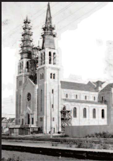
The cathedral under construction in August, 1913, with trolley tracks and a wooden sidewalk in front.
